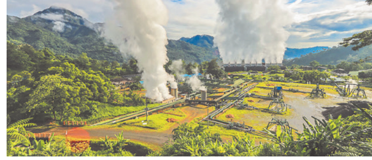
EDC's Palinpinon-1 geothermal power facility in Negros Island.
