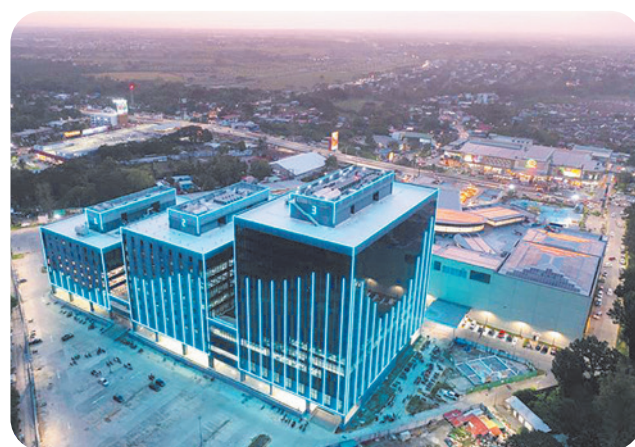
Cybergate Iloilo Towers. A business destination designed to enable productivity and steady expansion in Western Visayas.
