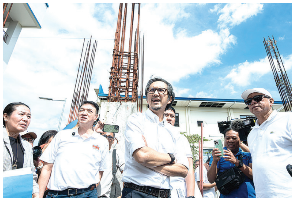
DPWH Secretary Vince Dizon, accompanied by Bacoor City Mayor Edwin Bautista and school officials, inspect the unfinished two-story building at the Responsible Village Leaders Learning Academy (REVILLA) High School in Bacoor City, Cavite on Feb. 3.
