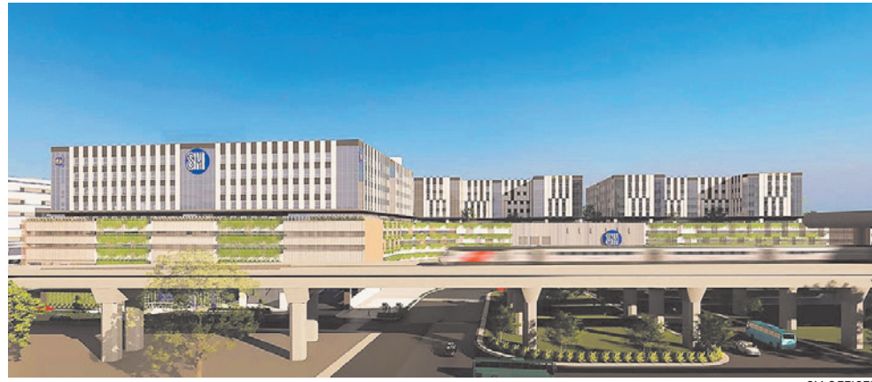
SM CLARK TOWERS integrates a future-ready workplace with an onsite transport hub for optimal accessibility.
