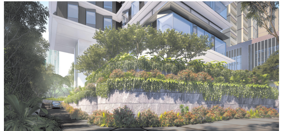
A private, landscaped approach creates a physical buffer from the surrounding streets, separating the development from the urban environment from the moment of arrival.
