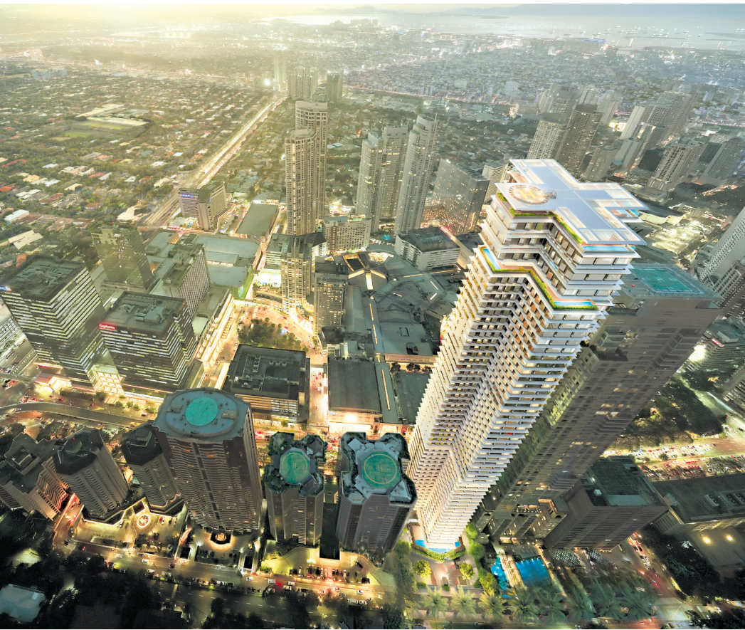
Deep horizontal fins on the façade provide essential shading and reduce solar gain, tailored for the tropical climate.
