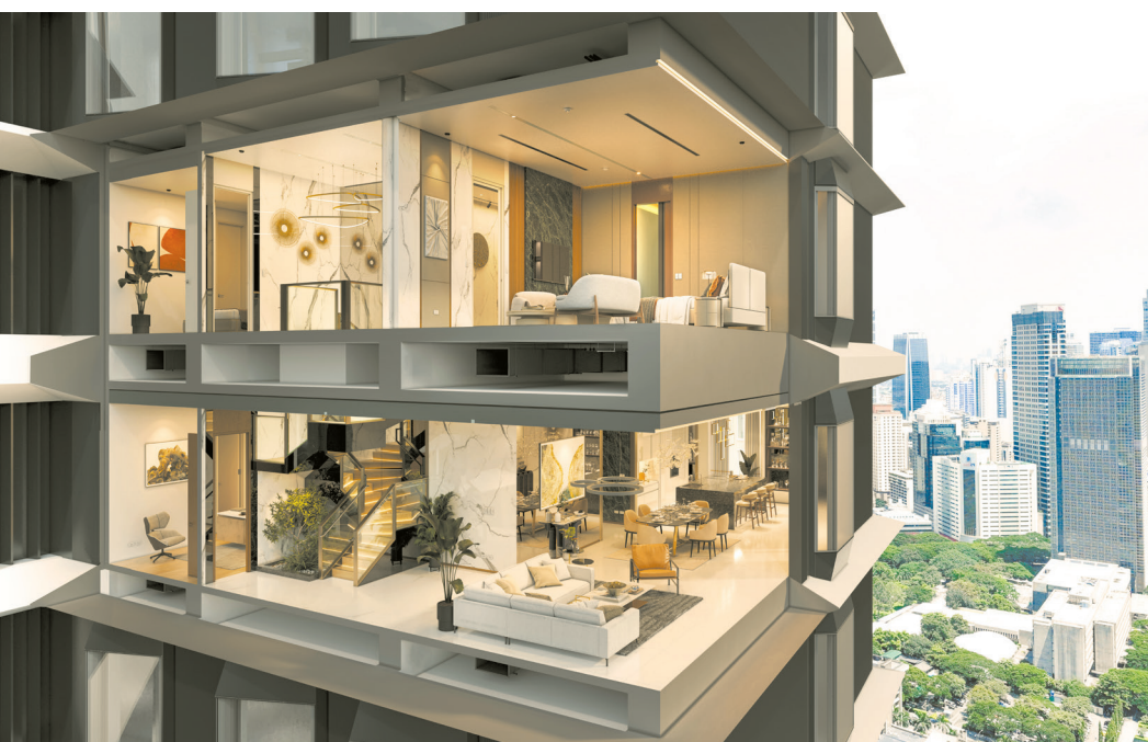
The double slab system allows rooms to expand or change function entirely, ensuring that reconfiguring a unit is a question of intent rather than structural intervention.
