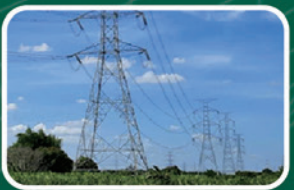
MARIVELES-BALSIK 500KV T/L COMPLETED: MAR 2022 COST: PhP4.44 BILLION
