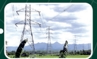
MINDANAO 230KV TRANSMISSION BACKBONE COMPLETED: NOV 2020 COST: PhP6.14 BILLION
