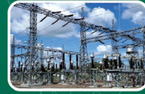
CALAMBA 230KV SUBSTATION COMPLETED: MAY 2021 COST: PhP1.21 BILLION
