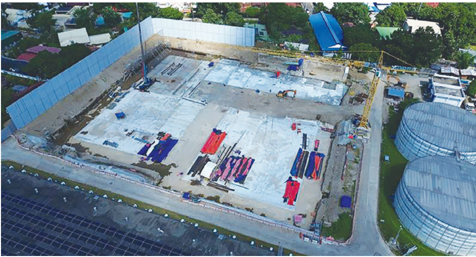
AN AERIAL VIEW of the ongoing demolition of the old San Juan Reservoir and the construction of the new 56-ML earthquake-resilient facility along N. Domingo Street in Quezon City.
