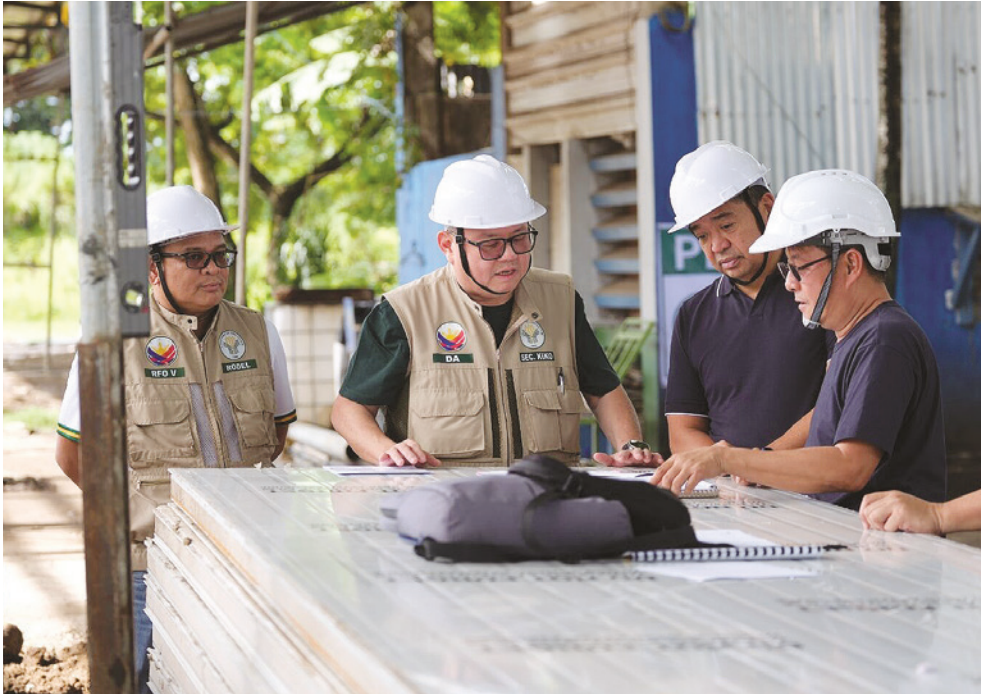
DA PRESS OFFICE AGRICULTURE Secretary Francisco P. Tiu Laurel, Jr. and Camarines Sur Governor Luis Raymund Villafuerte inspected the ongoing construction of a P500-million cold storage facility.
