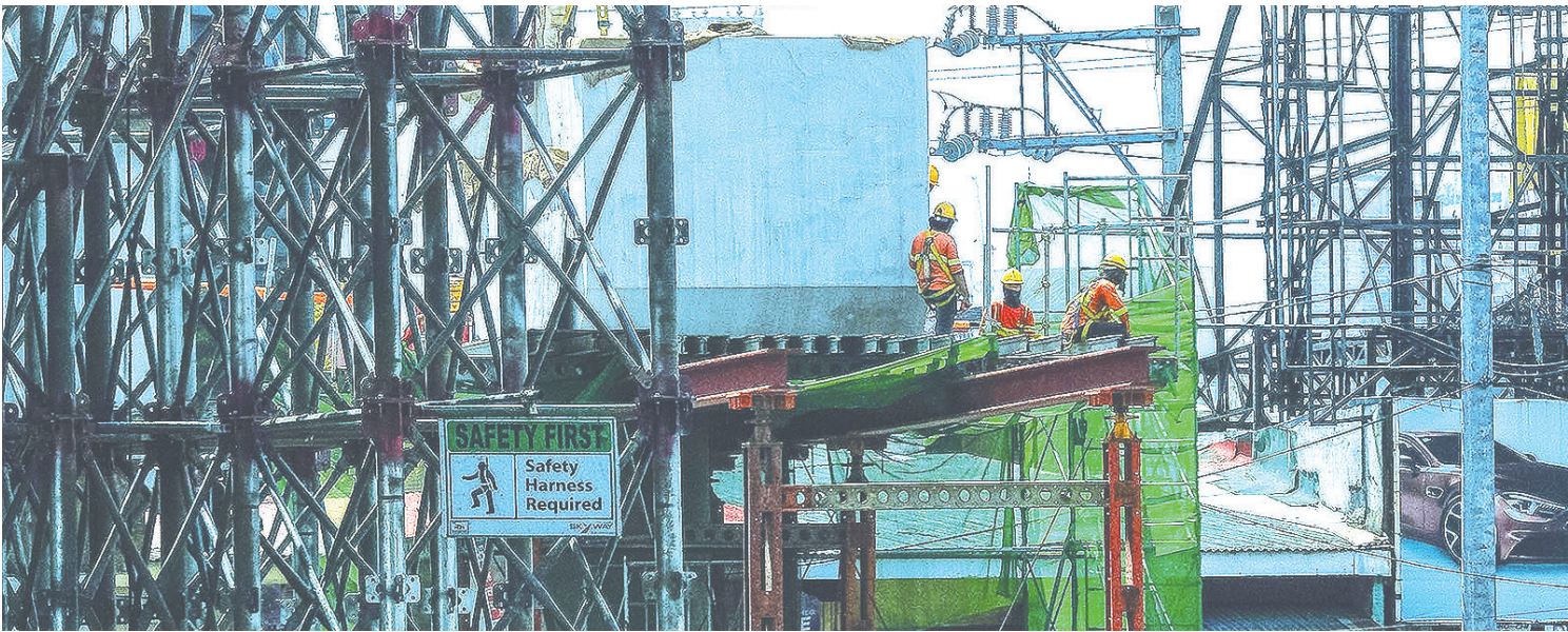
CONSTRUCTION WORKERS continue work on the Skyway project at the corner of Quirino Avenue and Osmeña Highway in Manila.
