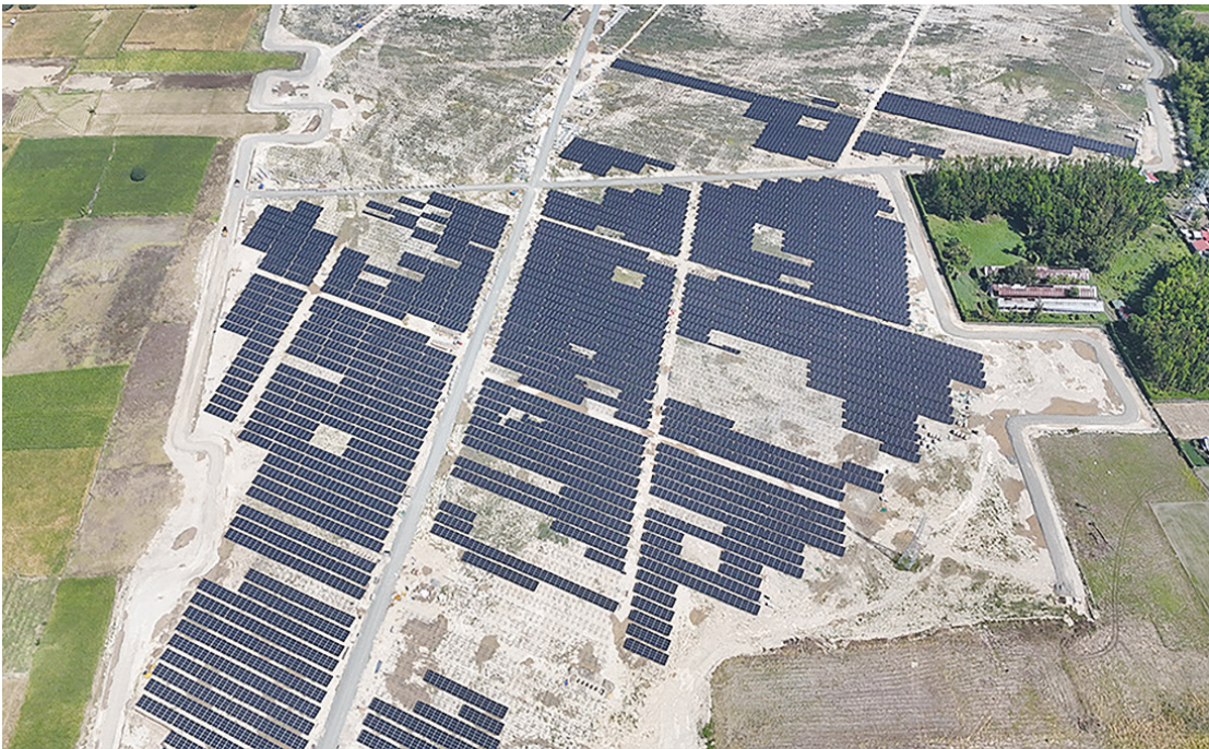
STA. BARBARA 1 Solar Power Project in Pangasinan
