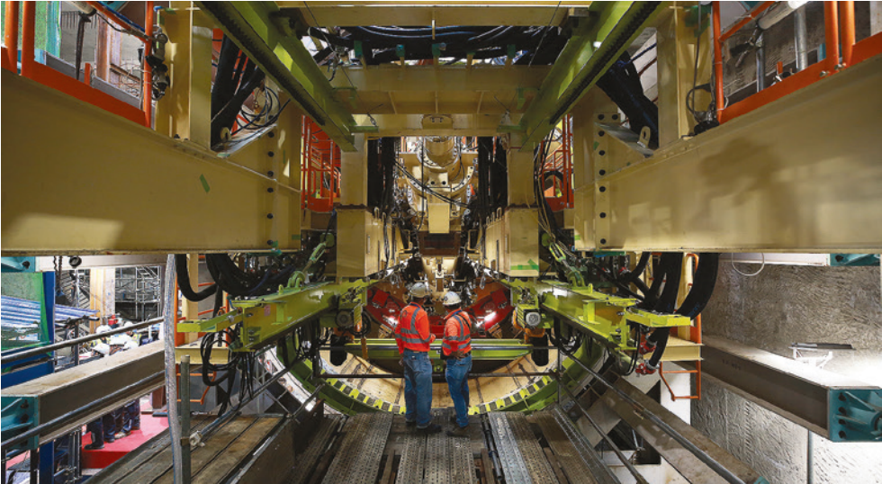
THE Tunnel Boring Machine at the Camp Aguinaldo station of the Metro Manila Subway Project in Quezon City on Jan. 16.
