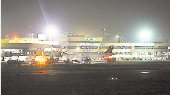
PHILIPPINE STAR/MIGUEL DE GUZMAN NEW NAIA INFRA CORP. Chairman Ramon S. Ang said the new terminal will add 36 passenger boarding bridges and accommodate 22 million passengers annually.
