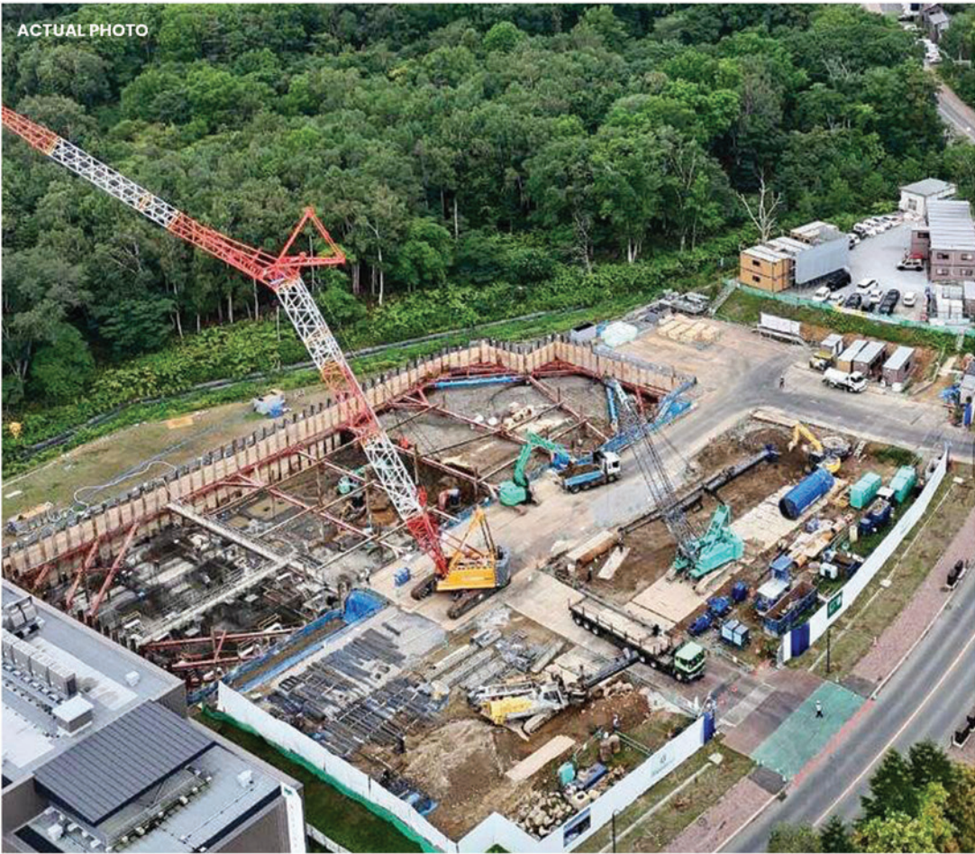
The 482-Room Hotel101-Niseko continues to progress nicely.
