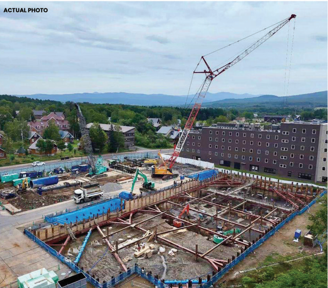
Very good weather now at the construction site in Niseko, Hokkaido, Japan.
