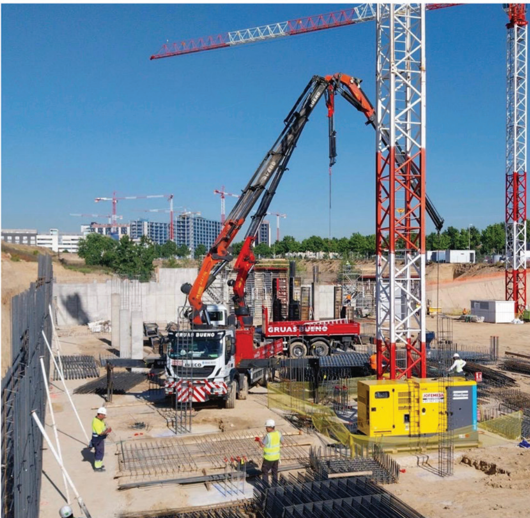
(Actual construction site photo of the 680-room Hotel101-Madrid Spain project)
