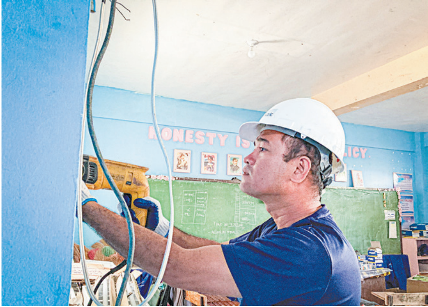
Rewired. Volunteer engineers of AboitizPower’s Visayan Electric have modernized the electrical wiring systems of 5,311 classrooms and school facilities, minimizing the risk of fire hazards and electrocution accidents.
