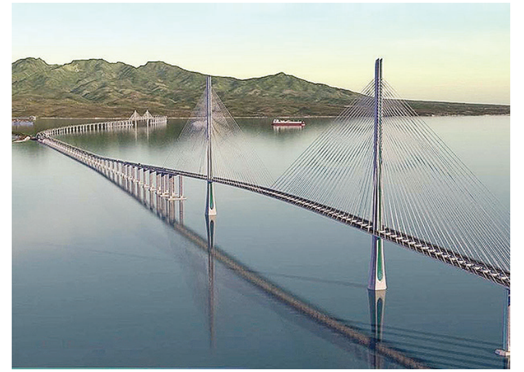
BATAAN-CAVITE Interlink Bridge
