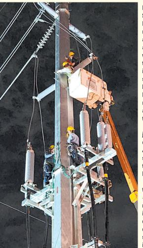
MERALCO **IMPROVES** SERVICE IN PASAY CITY -Manuel V. Pangilinan-led Manila Electric Company (Meralco) recently constructed a new 115 kilovolts (kV) line with a length of 2.1 kilometers to improve the reliability of its sub-transmission system in Pasay City. The PAGCOR 1-CBP1A 115 kV Line will also accommodate new customer applications and future load growth in the area.
