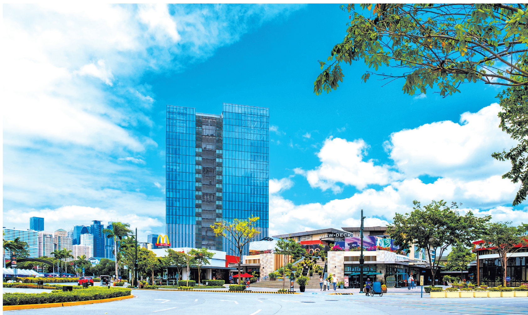
One Paseo inside ArcoVia City, one of 37 LEED-certified Megaworld office buildings in the country today, stands as proof of the company's continuing thrust to integrate sustainability within its township developments.
