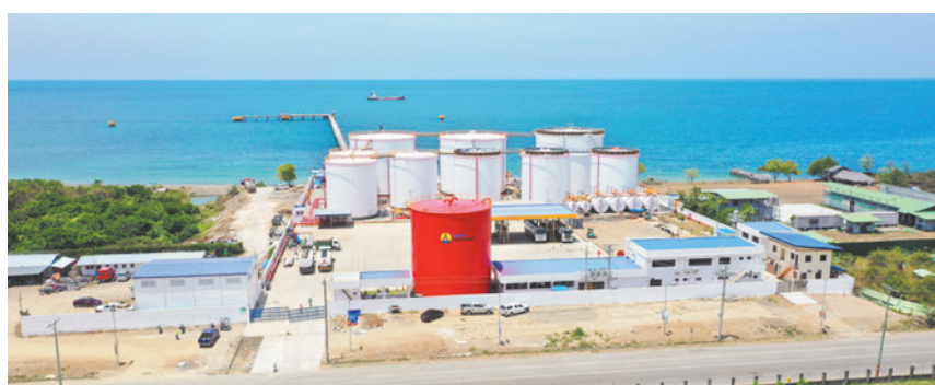
SEOIL ZAMBOANGA BULK TERMINAL
