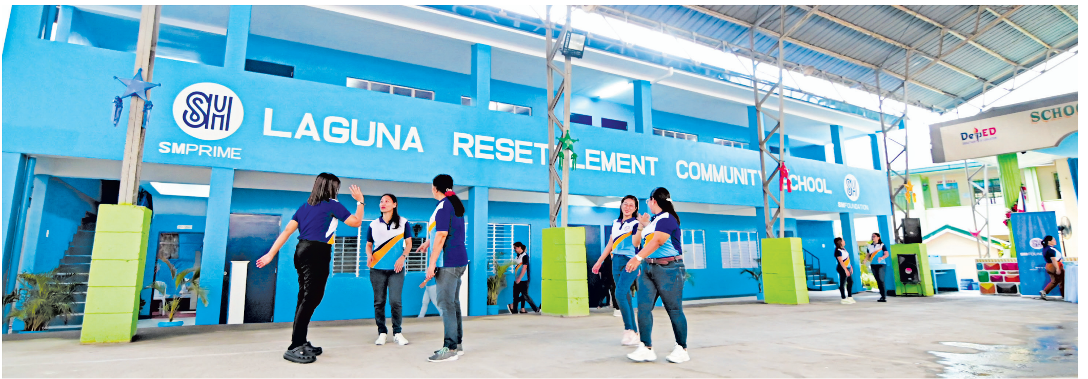
The new two-floor school building of Laguna Resettlement Community School (LRCS) features four fully equipped rooms with PWD-friendly facilities.
