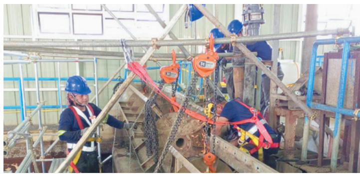
THE west zone water concessionaire's intended improvement is in response to the worsening quality of the raw water from Laguna Lake.
