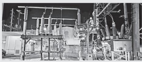
Meralco recently upgraded its Zapote Substation located in Barangay Elias Aldana, Las Piñas City with the installation of one (1) three-phase 115-kV power circuit breaker, two (2) three-phase 115kV disconnect switches, and various protection and control equipment. This is in conjunction with NGCP's installation of a fifth 300-MVA power transformer bank in its Las Piñas Substation. This aims to provide additional capacity to serve the increasing power demand in Pasay City, southern parts of
