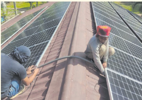
Solar panels being installed at Pueblo de Oro Golf & Country Club
