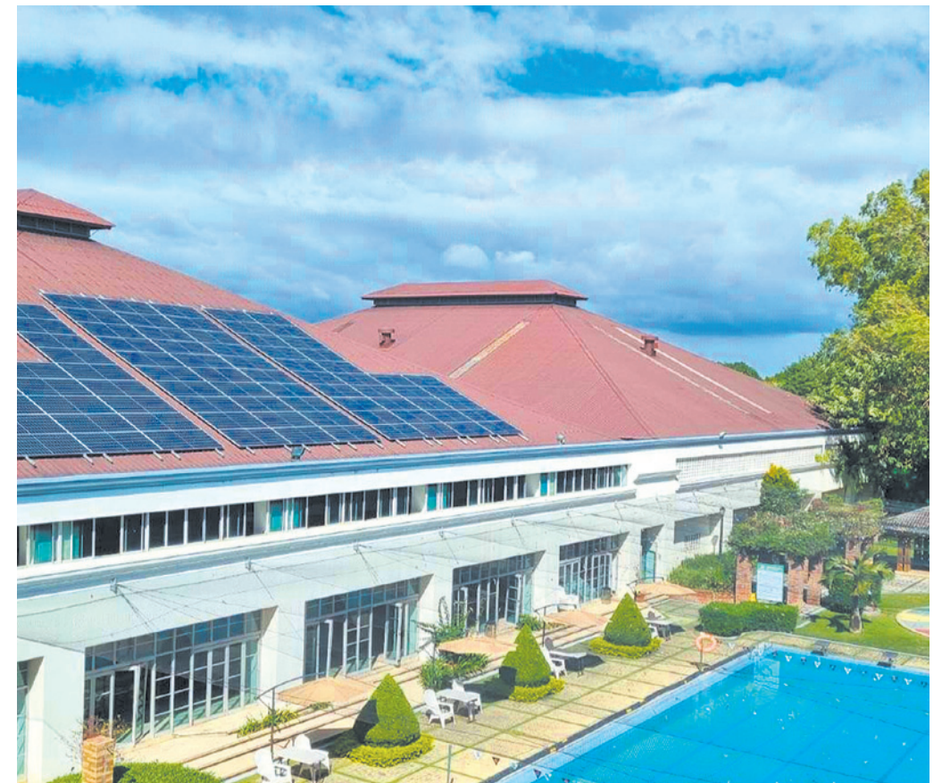
Spectrum's partnership with The Orchard involved a solar rooftop project with a capacity of 99.9 kilowatt-peak installed at the latter's sports and leisure facility in Dasmariñas, Cavite.
