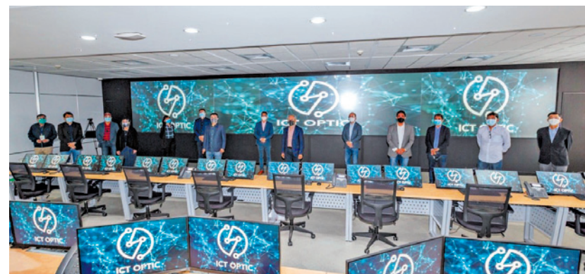
Meralco executives showcase the new ICT OPTIC, a new state-of-the-art facility that aims to reduce unplanned downtime of critical ICT systems, increase productivity of employees, and enhance service delivery to customers.
