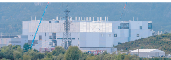
CONSTRUCTION of the new chip factory of Infineon Technologies Austria AG
