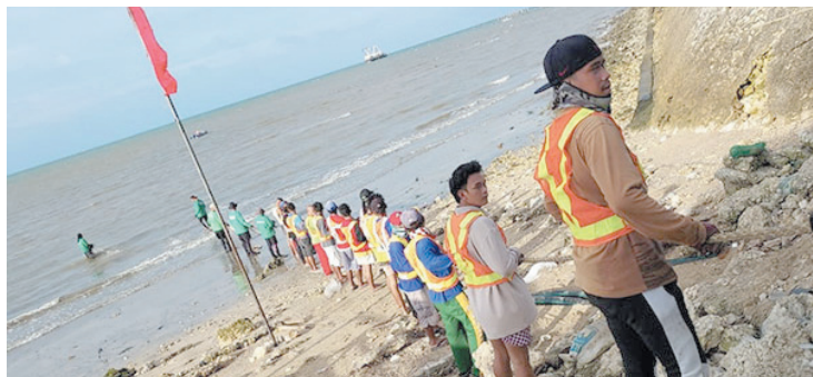
LANDING of Globe's submarine fiber cable in Placer, Masbate.
