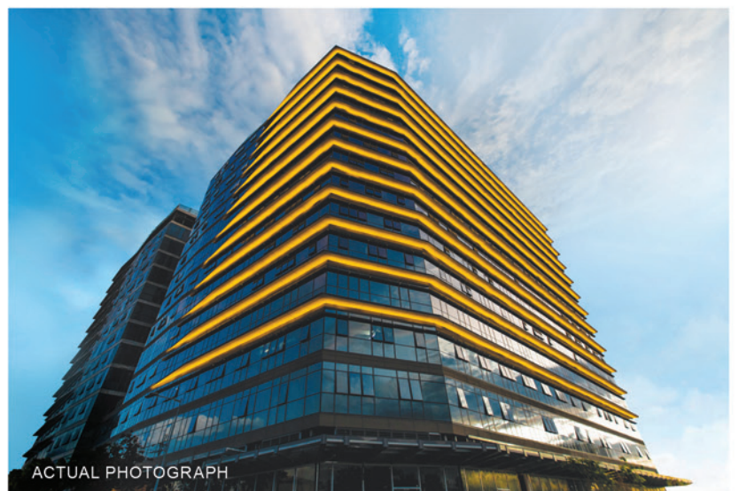
The Savva Financial Center (ARCA South, Taguig). The first premium green office building in one of the most connected central business and lifestyle districts of Metro Manila.
