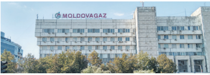
MOLDOVAGAZ headquarters on Albişoara st., Chişinău
