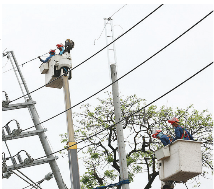
WORKERS FIX an electric line in Payatas, Quezon City, March 13.
