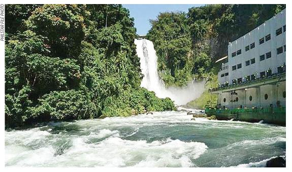
consists of seven hydropower plants originally rated at 1,001 megawatts (MW), though only 600 to 700 MW are available due to the inefficiency of the aging facilities.
