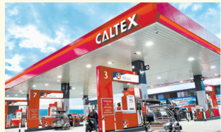
The newly opened Caltex station in Barangay Masipit, Calapan City, Oriental Mindoro is ready to serve quality fuels and lubes to locals and travelers alike.
