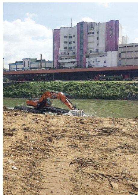
AMPHIBIOUS EXCAVATOR operating to dredge heavily-silted portions of Marikina River. DPWH.GOV.PH
