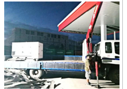
Ten generator sets were deployed through F2 Logistics from Davao to Cebu.
