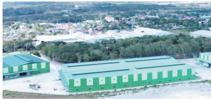
COMPLETED CentralHub in Tarlac
